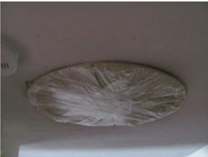
House attic sealed closed
