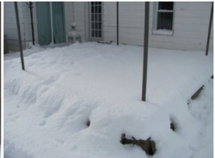
Deck covered with snow and no access underneath
